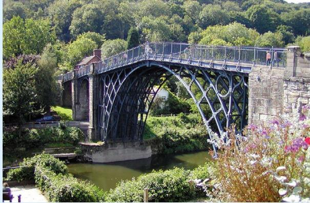
Spanning 100 feet at 60 feet above the water level, the bridge across the River Severn at **Ironbridge** in Shropshire, opened on New Year's Day 1781, was the world's first cast iron arch bridge. With no precedent for the design, construction was based on traditional carpentry experience – the 800 individual castings of 12 basic components were fastened together using familiar wood-working techniques such as mortise and tenon and dovetail joints rather than welds, nuts and bolts or rivets.
