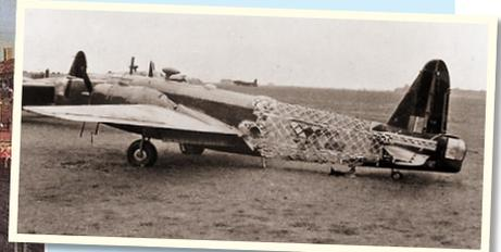
The geodesic construction of its fuselage – devised by **Barnes Wallis** of bouncing bomb fame – allowed the **Vickers Wellington** bomber to survive terrible damage while remaining airworthy. A propaganda exercise in October 1943 saw a **Wellington** assembled in 23 hours 50 minutes and airborne 58 minutes later.
